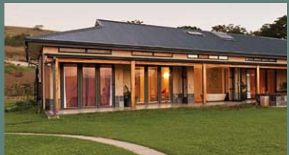
The completed House Kahler took just five months to complete using the LSF building system
