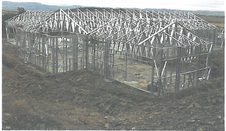
The light steel frame structure of the house.
